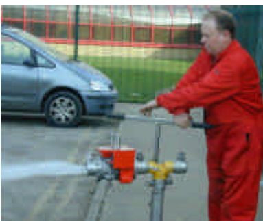
Hydrant flow test in progress
